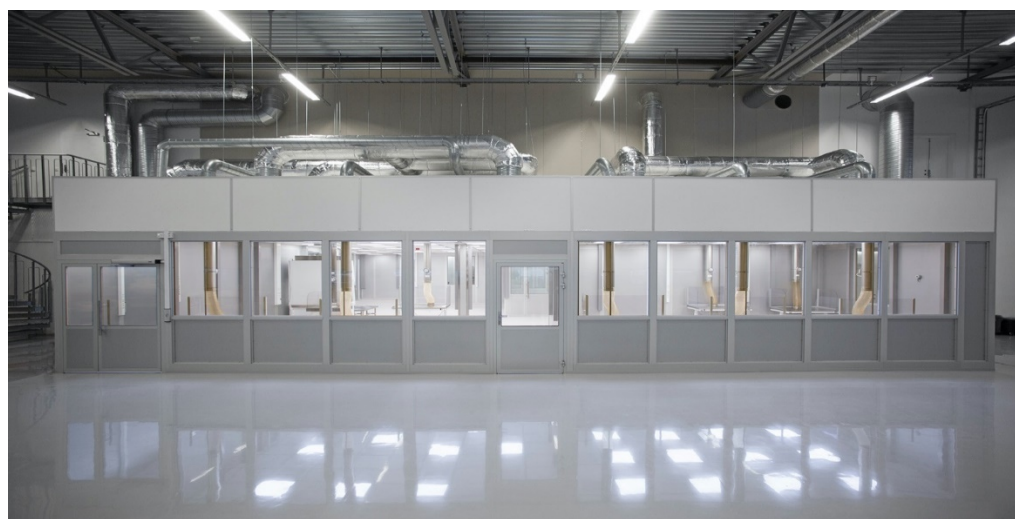
Cleanroom at APL
